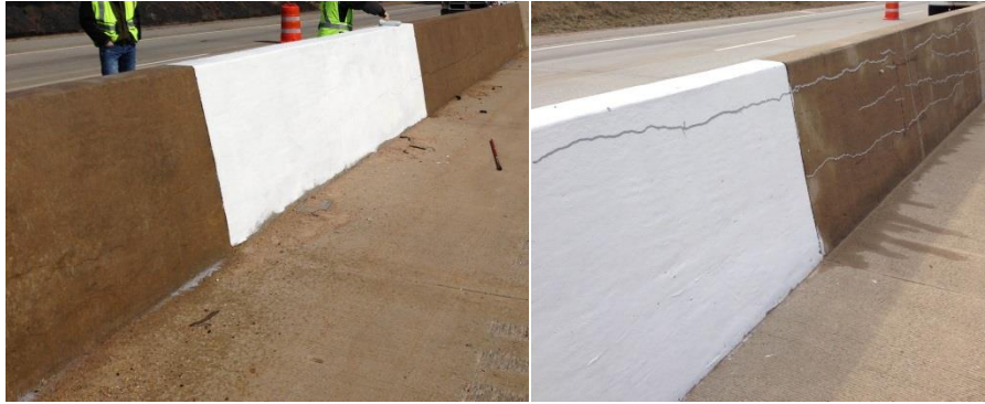
Figure 2.10. Application of surface treatment (left) and crack sealant (right). Pictures used with permission from Richard Deschenes.
